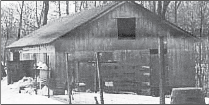
The finished barn.
